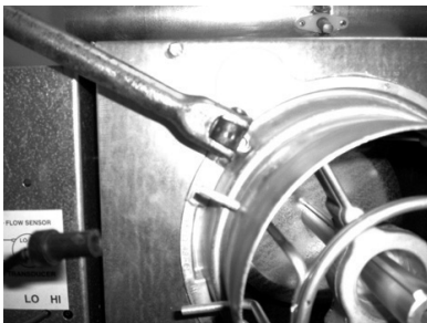
Figure 4. Remove pneumatic tubing
